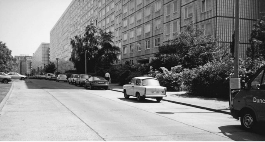
Massiveness was one hallmark of the Soviet planning style. This is a Soviet-era housing project in the former East Berlin.
