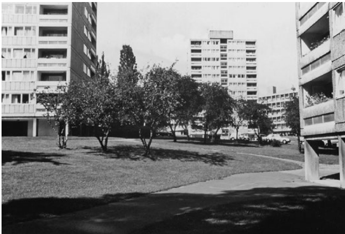
Le Corbusier's "Voisin" plan for Paris 1922–1925 (top). Building very high would permit extreme population density while leaving 95 percent of the land vacant. Although never built, this plan exerted enormous influence on design, for both better and worse, in many countries. Below is the planned community of Roehampton in Great Britain. Note the Le Corbusier influence in the large amounts of interior open space and the use of columns referred to as pilote .
